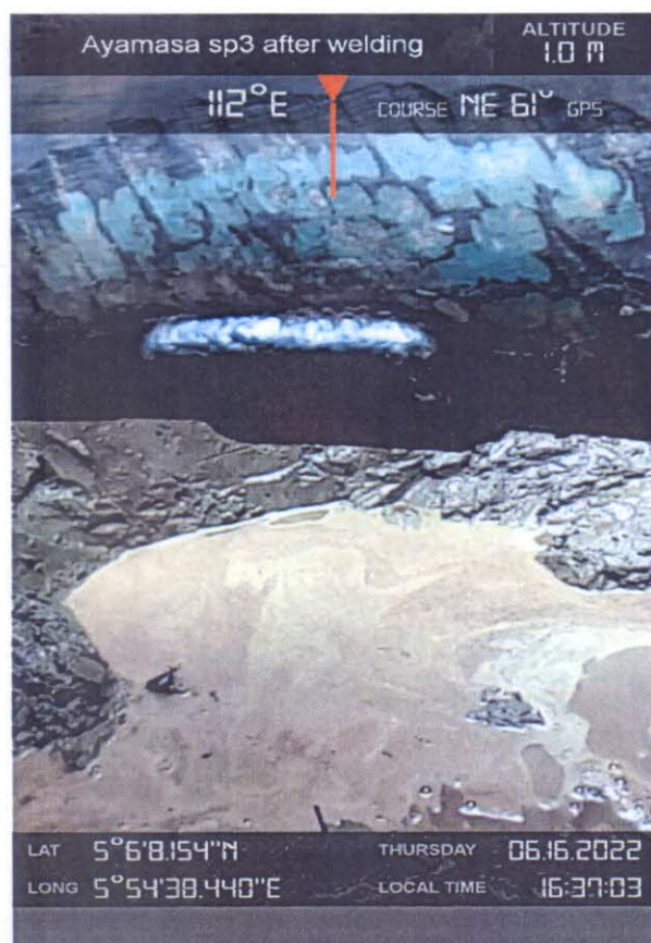
Fig: 3. During Repairs
